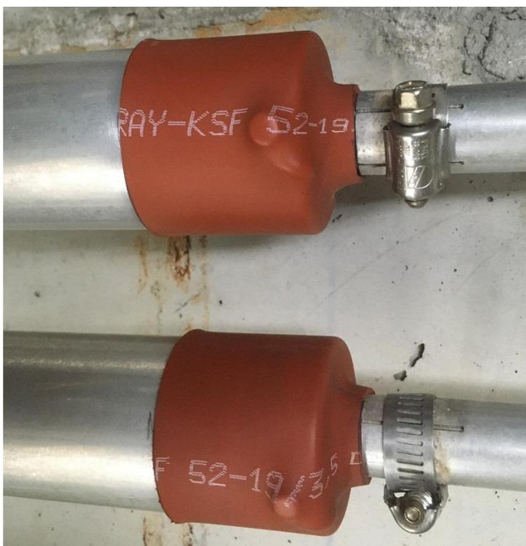
**FOTO-11 TERMORETRÁCTIL INSTALADO**
